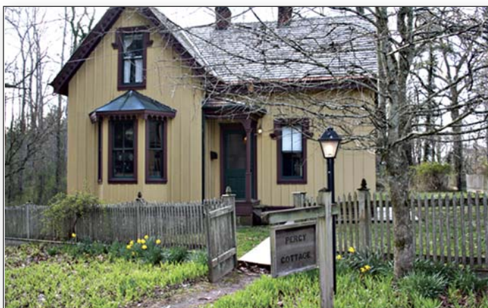
Percy Cottage rents out an upstairs two-bedroom suite. The downstairs rooms are used for office space.
