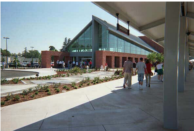
This new station in Bakersfield, CA was funded by the State of California.
