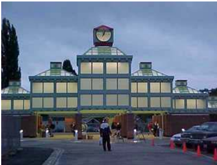
Sounder-Auburn Station. New passenger stations should be both attractive and cost effective.
