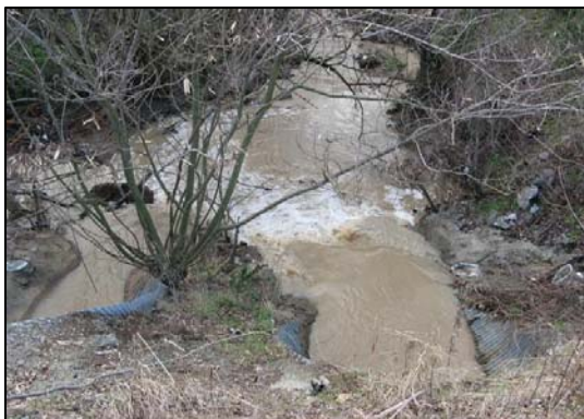
Looking Downstream at STR-4 from SR 22
