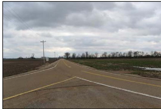
Looking South at SR 22 from End of Project
