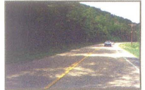
Phase II, near Old Hills Creek Road (looking west)
